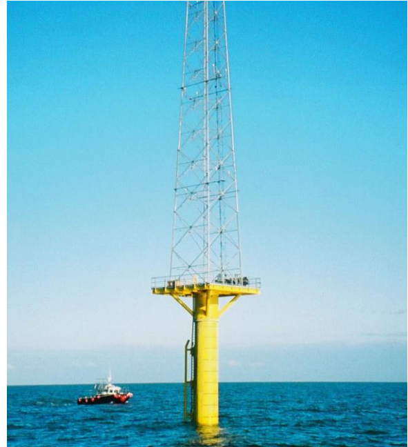
Figure 1: 70m met mast in the North Sea
